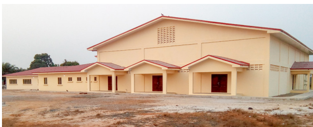
The new RICE building
