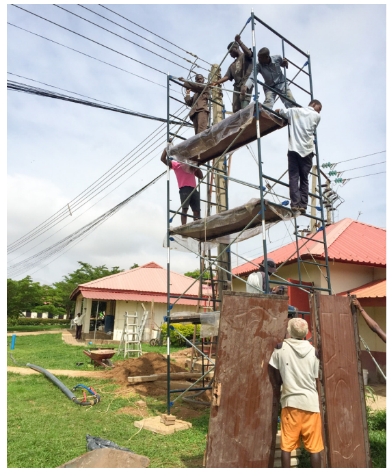
Power cable being replaced
