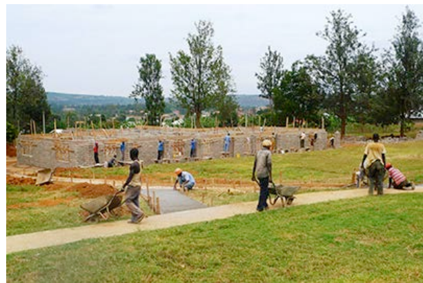
New Junior Secondary School being built
