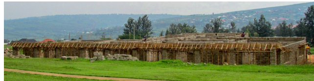
Ready for the roof
