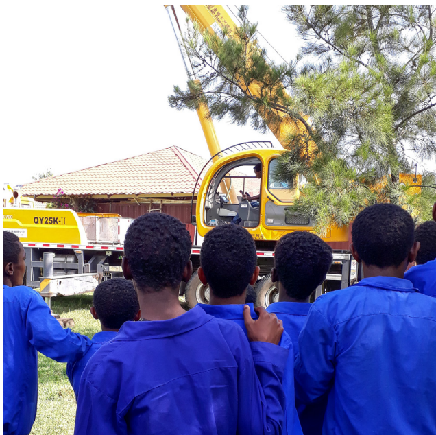
Watching the container being delivered
