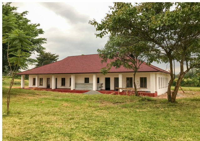
Progress as of August 7
