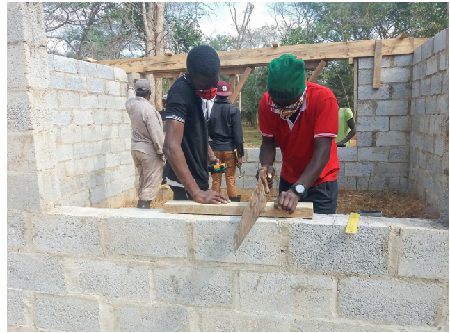
Building a chicken house
