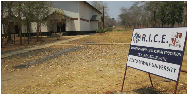
New sign in front of the RICE building
