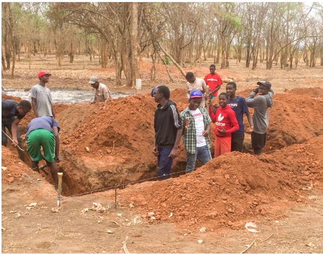
Digging the foundation of the chicken house
