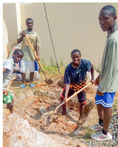
Young men in Liberia helping with construction during the COVID lock-downs.
