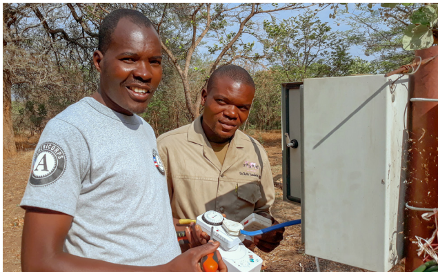
Plant manager and assistant working on pump for the water tanks
